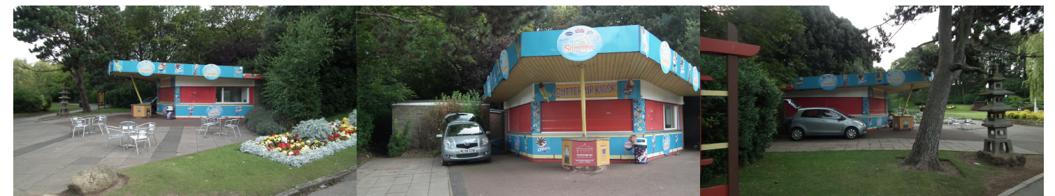
photos of the existing buttercup kiosk
